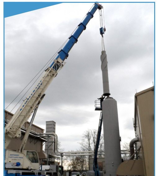
Exhaust Stack Install
