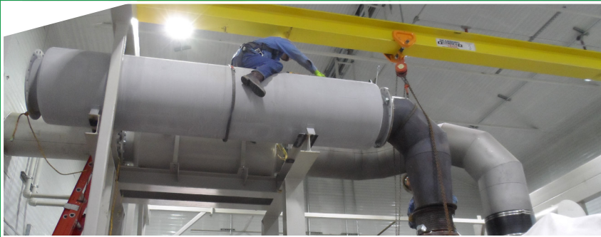
Engine Resonator Install
