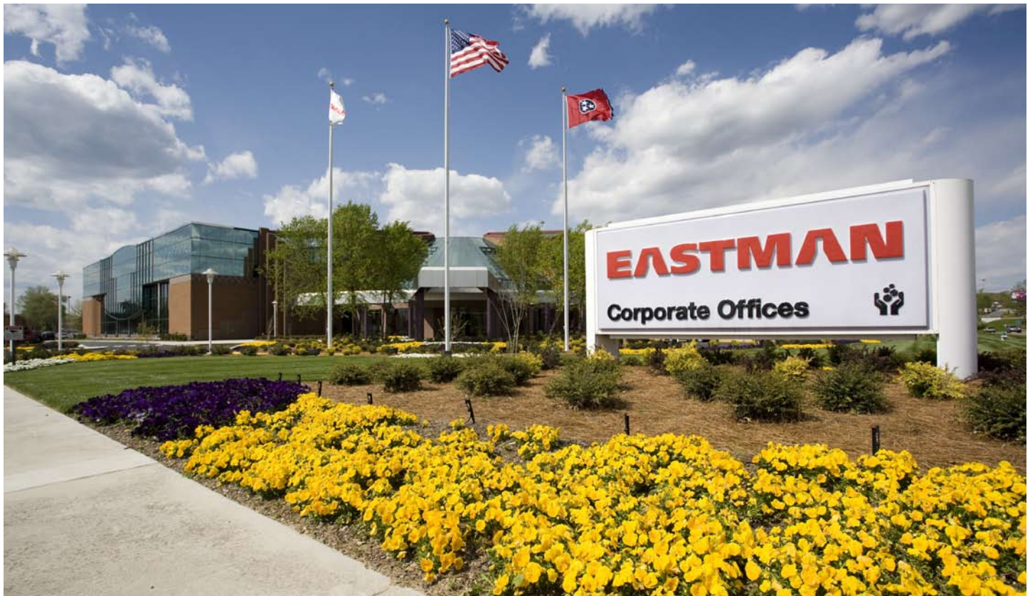
The corporate headquarters of the Eastman Chemical Company in Kingsport, Tennessee in the USA.
