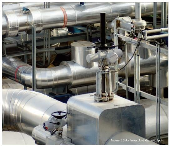
installations, Pakscan can operate a loop of up to 20 kilometres in length without any deterioration in communication performance or the need for repeaters. This has enabled over one hundred actuators at each Andasol site to be controlled and monitored with a single bus loop. Each loop is supervised by a Pakscan P3 120 channel master station, which provides the communication interface with the plant's control centre.
